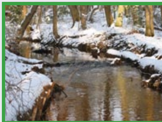
Completed installation showing weir and streambank fiber logs
