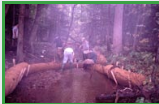
Installing coir fiber logs cross weirs
