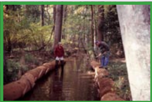
Installing coir fiber logs along stream bank
