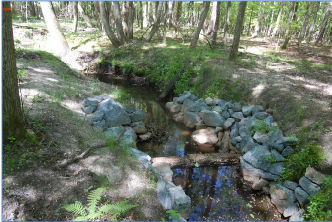
Figure 20: Looking downstream at modified log vane #1. Notice deposition along banks. (April 2010)
