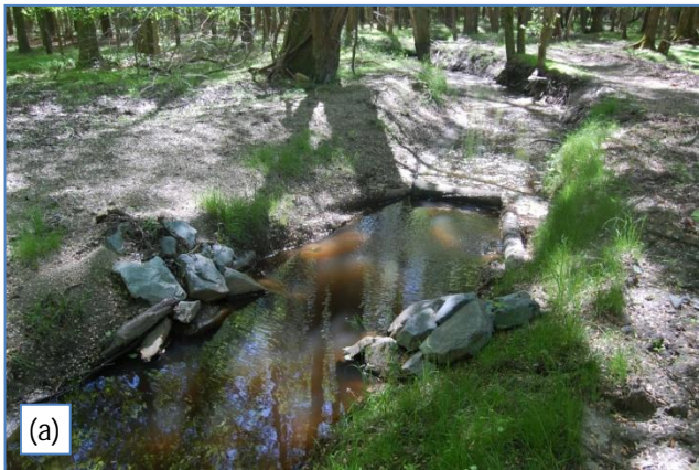
Figure 15: Log vane #6 (a. looking upstream, b. looking downstream), notice the significant amount of deposition in the floodplain. (April 2010)
