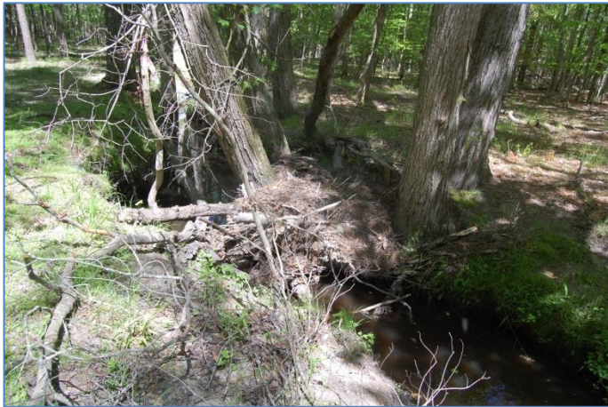
Figure 18: Debris jam between log vanes #2 and #3. Notice the height of debris above the flow. This indicates the flows are frequently overtopping the banks. (April 2010)
