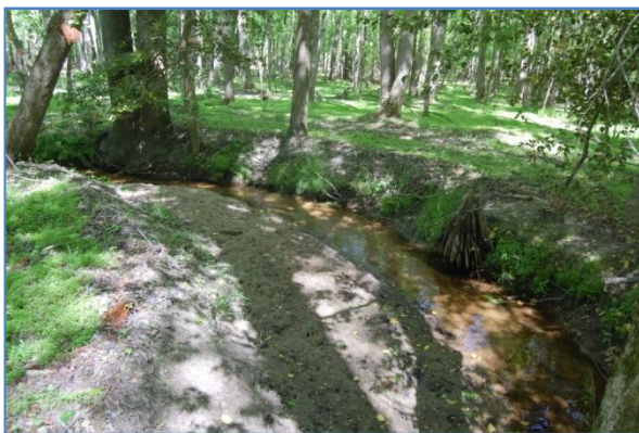
Figure 16: Bar formation and channel deposition between log vanes #6 and #7 (April 2010).
