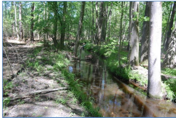
Figure 16: Bar formation and channel deposition between log vanes #6 and #7 (April 2010).
